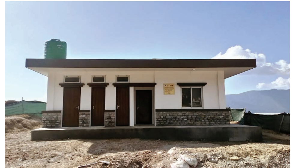
Newly constructed Barpak Women's Community Center in Barpak, Gorkha
