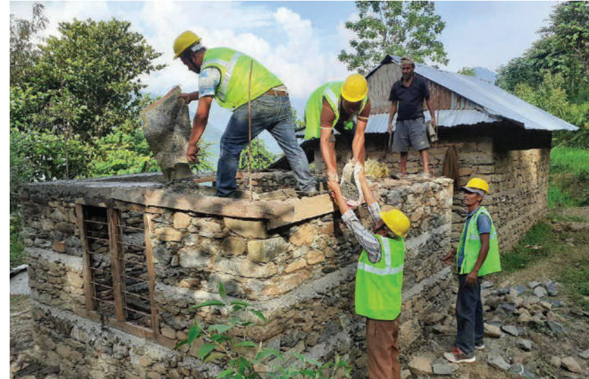
Masons at work in Sindhupalchowk
